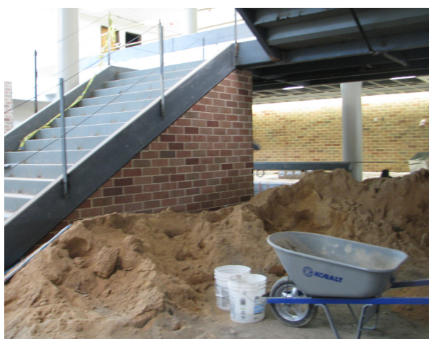
Current construction on East's upcoming lobby and new wing.
